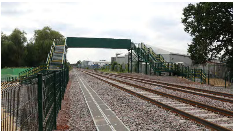
The first section of track to be commissioned near Bicester Fringe
